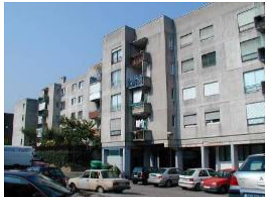
late 70-ties, cast in place reinforced concrete “self standing” blocks, low TI
