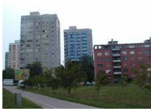
late 50-ties, masonry, no TI, high rise building
