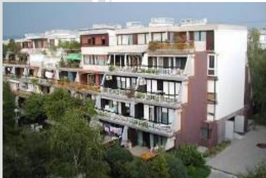
late 70-ties, reinforced concrete, pre-cast large panels; low TI, thermal bridges, envelope elements, masonry, GF + 4 storeys
