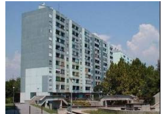
late 70-ties, concrete high multi-story buildings with pre-cast large panel envelope elements
