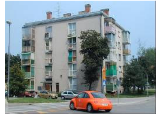
early 60-ties, masonry, no TI, self-standing building
