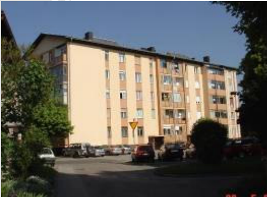
Non-renovated apartment house Sisenska 42-44 in Ljubljana. IR thermography detected cold bridges in the envelope: (joints of concrete panels).
