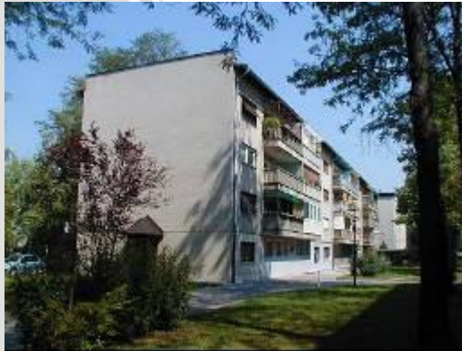
50-ties, masonry, no TI, GF + 3 storeys
