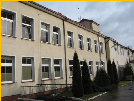
Hospital in Kwidzyn (photo by BAPE)
